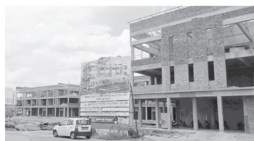
Shophouses currently under construction, adjacent to Star Mega Mall, Sibuan
