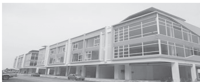
IBRACo's Tabuan Tranquility Commercial Centre at Stutong nearing completion
