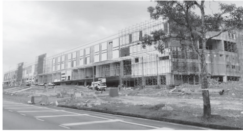
MYDIN under construction at Tiya Vista, Petra Jaya, Kuching
