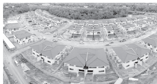
Rivervale Residences at Stutong developed by MIs CMS under construction
