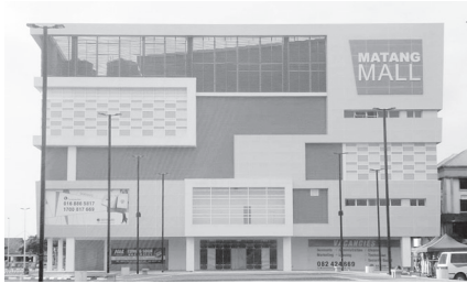
The newly completed Matang Mall, Kuching
