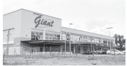
Newly completed Giant superstore at Petra Jaya, Kuching
