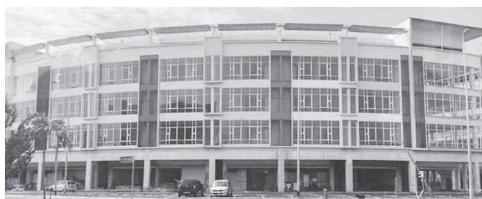
Newly completed Chayi Goldland at Jalan Stutong, Kuching
