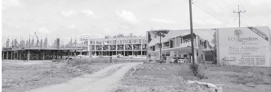
Eco Garden Residence sited opposite Sibujaya Township currently under construction
